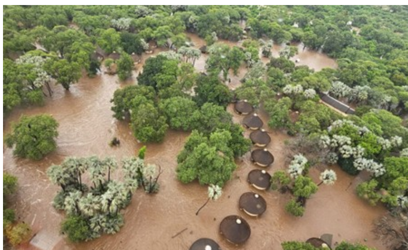
Figure 1. Flooding at the Kruger National Park, Letaba, in January 2026 (Source: Nordling, 2026).
